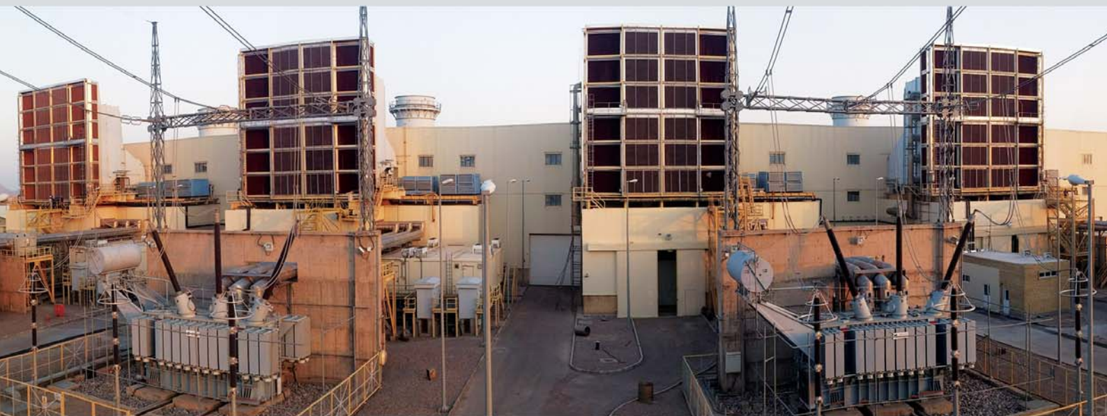
Media Evaporative coolers at Kaveh CCPP, Iran (2015)
