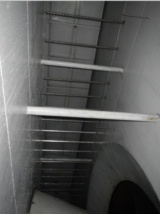
SPRAY AT BELLMOUTH OF THE COMPRESSOR
